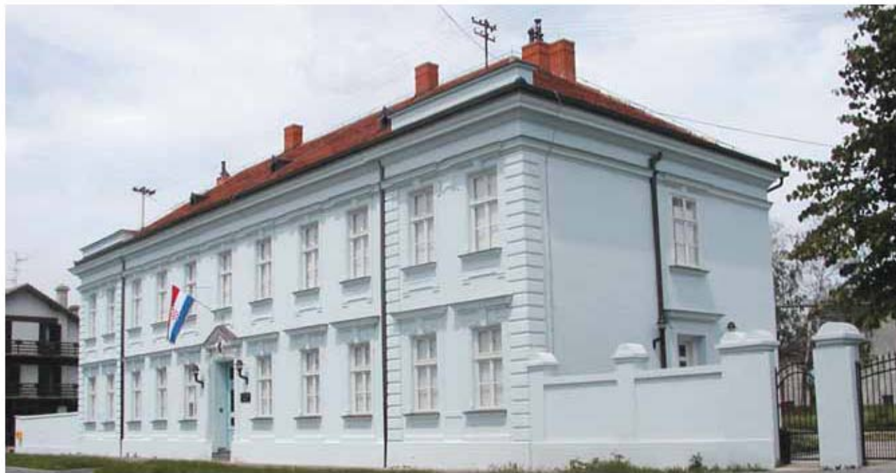
Zgrada u kojoj je danas smješten Muzej Đakovštine The building in which the Museum is currently located Das Gebäude in dem sich das Museum heute befindet
